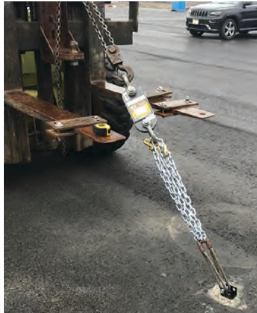
PULL TEST USING FORKLIFT
