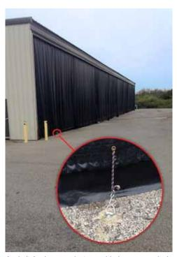
Asphalt Anchors products provided an economical solution to a windy problem for United Building Specailties of Auburnville, Florida. The anchoring system effectively anchored tarp walls to an asphalt lot for a temporary building to protect exotic lumber species from the harsh Florida elements.
